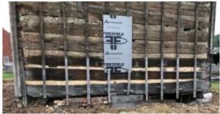
Detail of size of logs, notching and 19th century chinking, east elevation
