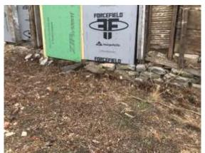
Debris, dirt at the original entrance, impacting stone foundation
