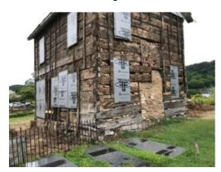
This image shows the historic west and north elevations. Note the interior chimney, a very unique feature of the building. Also note where it is located on a sligt grade, a typical feature of Pennsylvania log construction of the late 18<sup>th</sup> century.
